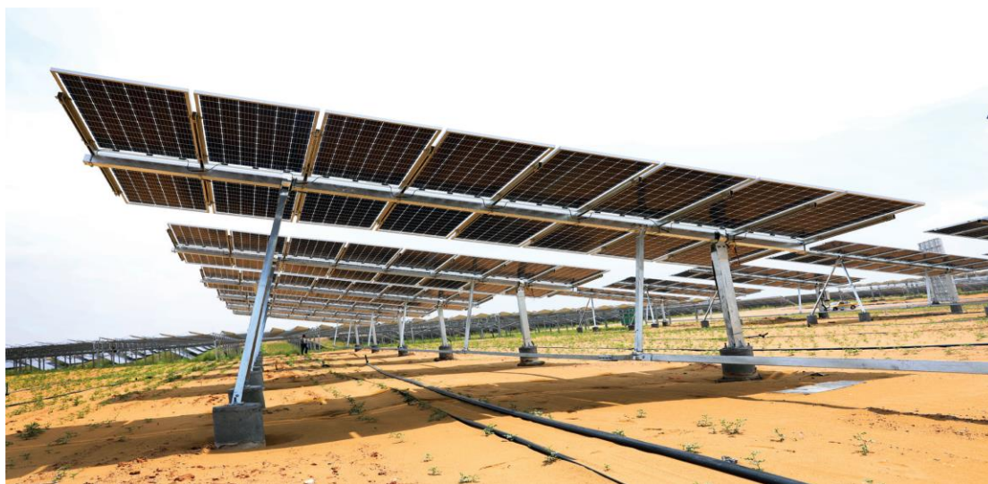
Figure 11 Sketch Map of Installation of Bifacial Module
