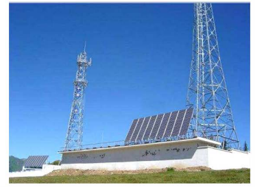
Communication base station, etc.
